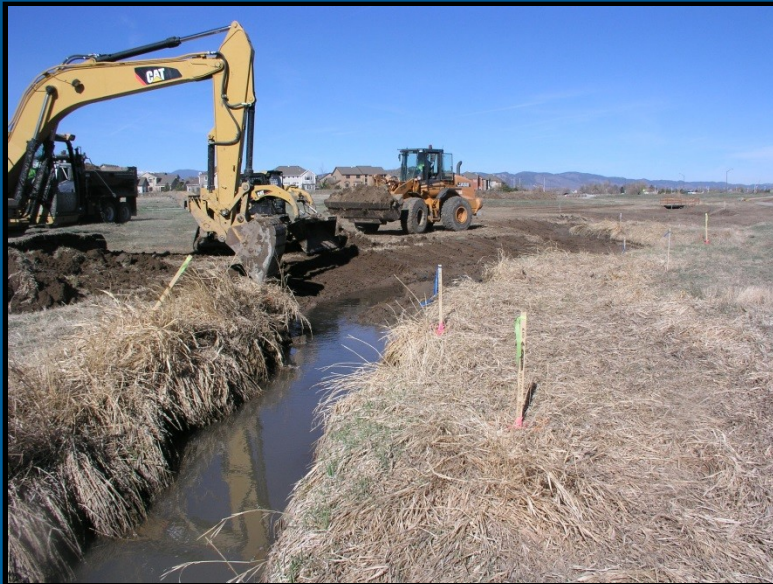
April 2012 McClellands Creek – During restoration
