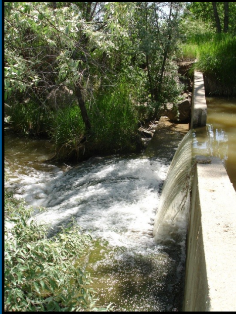
Irrigation Diversion Structure
