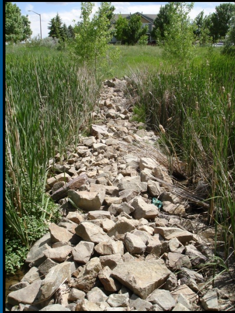
Grade Control Structure
